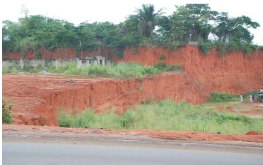
Plate 1. Sand excavators and excavated land in Atan community which threaten quality of life
